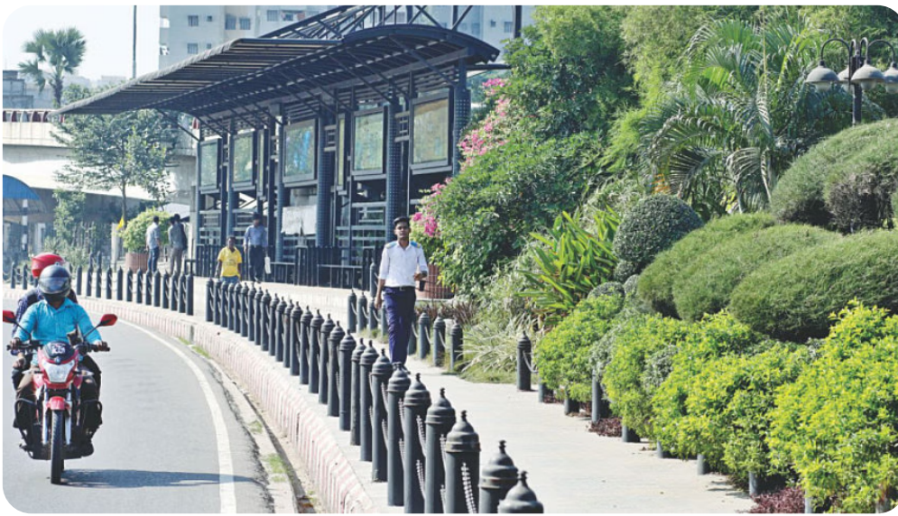
A shed for commuters on a tidy footpath on Airport Road. Photo: Prabir Das/Palash Khan
